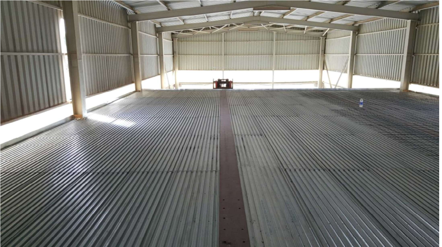
HYBRID STRUCTURE (HOT ROLLED AND COLD FORMED STEEL WITH LEWIS ® FLOORING)
