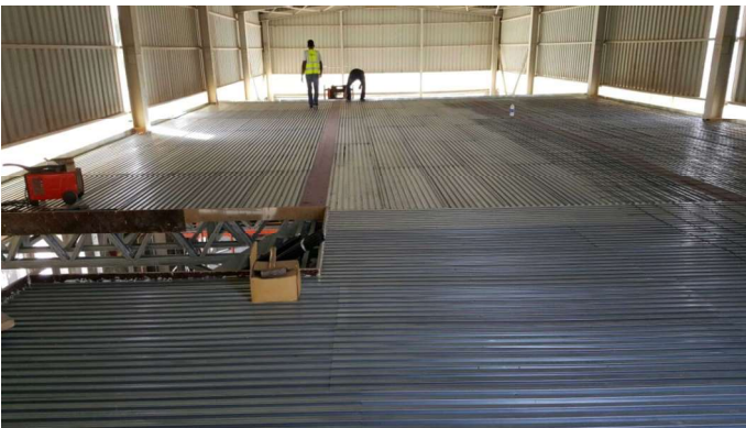
HYBRID STRUCTURE (HOT ROLLED AND COLD FORMED STEEL WITH LEWIS ® FLOORING)
