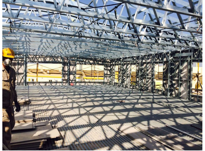
HYBRID STRUCTURE (HOT ROLLED AND COLD FORMED STEEL WITH LEWIS ® FLOORING)
