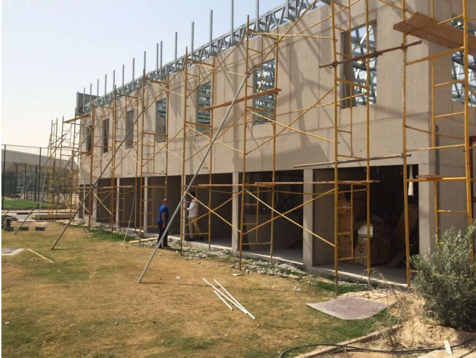
HYBRID STRUCTURE (HOT ROLLED AND COLD FORMED STEEL WITH LEWIS ® FLOORING)
