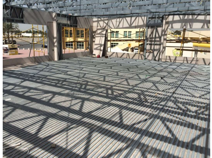
HYBRID STRUCTURE (HOT ROLLED AND COLD FORMED STEEL WITH LEWIS ® FLOORING)
