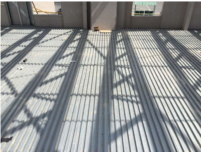
HYBRID STRUCTURE (HOT ROLLED AND COLD FORMED STEEL WITH LEWIS ® FLOORING)
