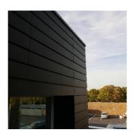
elZinc Graphite® harmonizes perfectly with other building materials. **elZinc Graphite®** is rolled architectural titanium zinc pre-patinated to a dark grey colour which is very similar to natural slate. This finish is produced after the surface has undergone a non-polluting phosphating process.
